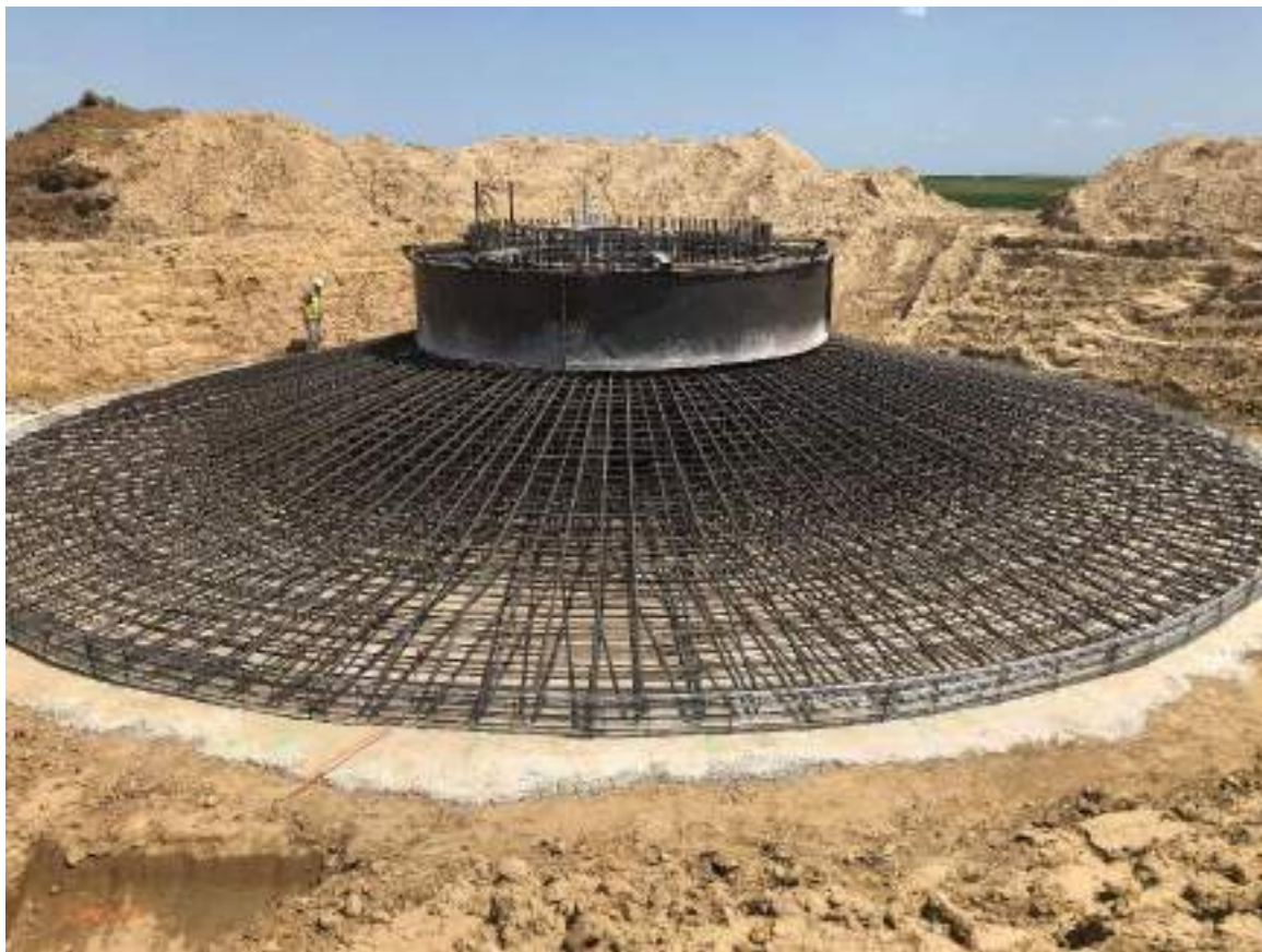
Figure 7: Wind turbine foundation in construction
