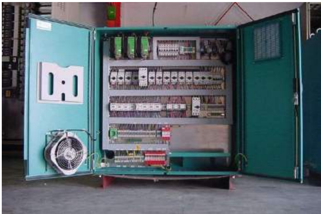
Figure 9: control circuitry for a wind turbine.
