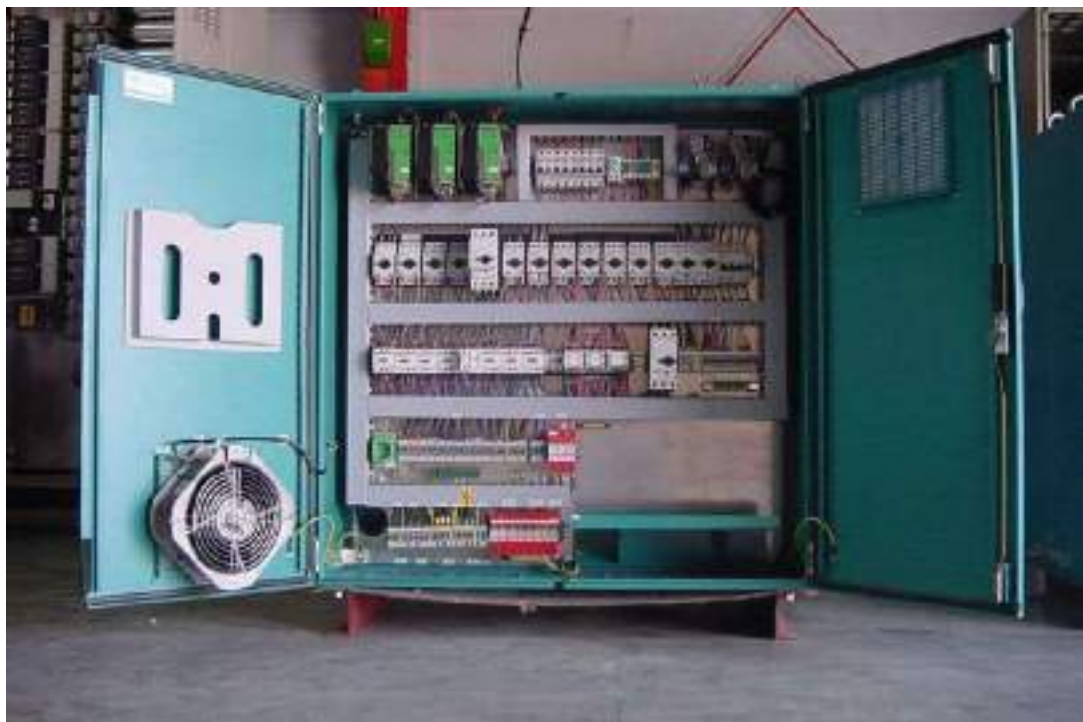
Figure 9: Control circuitry for a wind turbine.
