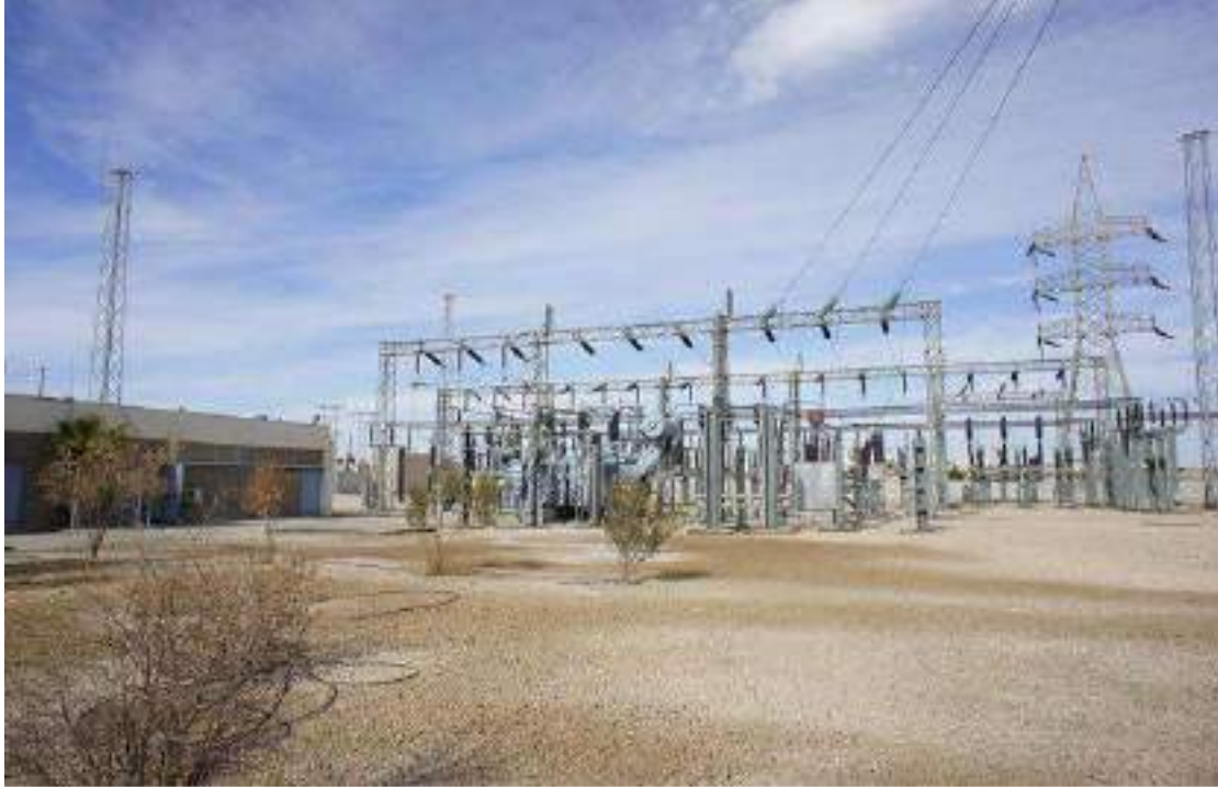
Figure 11: Typical 33/132kV Substation
