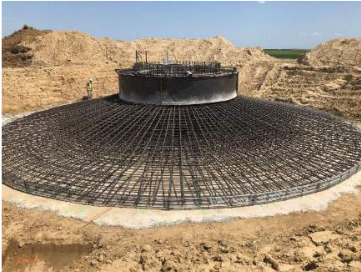
Figure 7: Wind turbine foundation in construction
