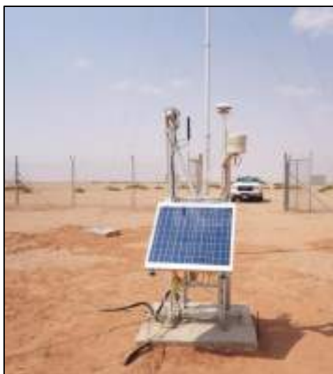
Figure 4-5 Meteorological Station in Saad Site
