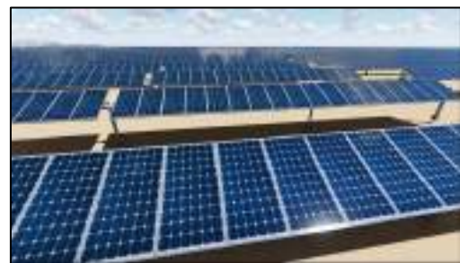
Single-axis tracking system
