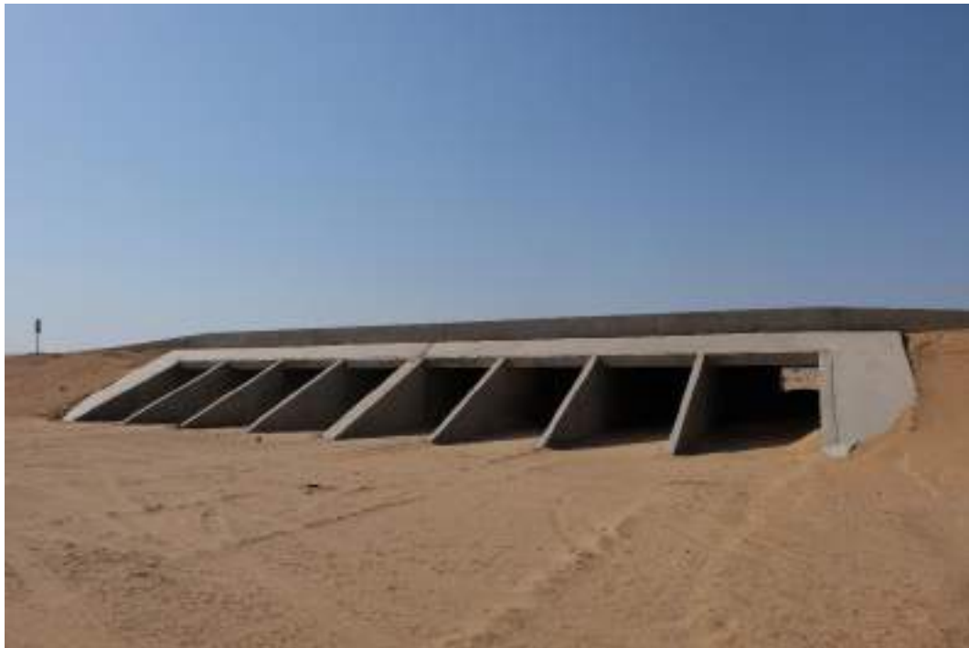
Figure 2-15: Typical culvert under a road
