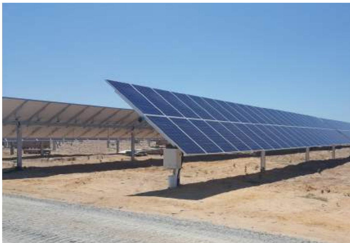
Figure 2-7: Example of solar PV modules mounted into strings on frames
