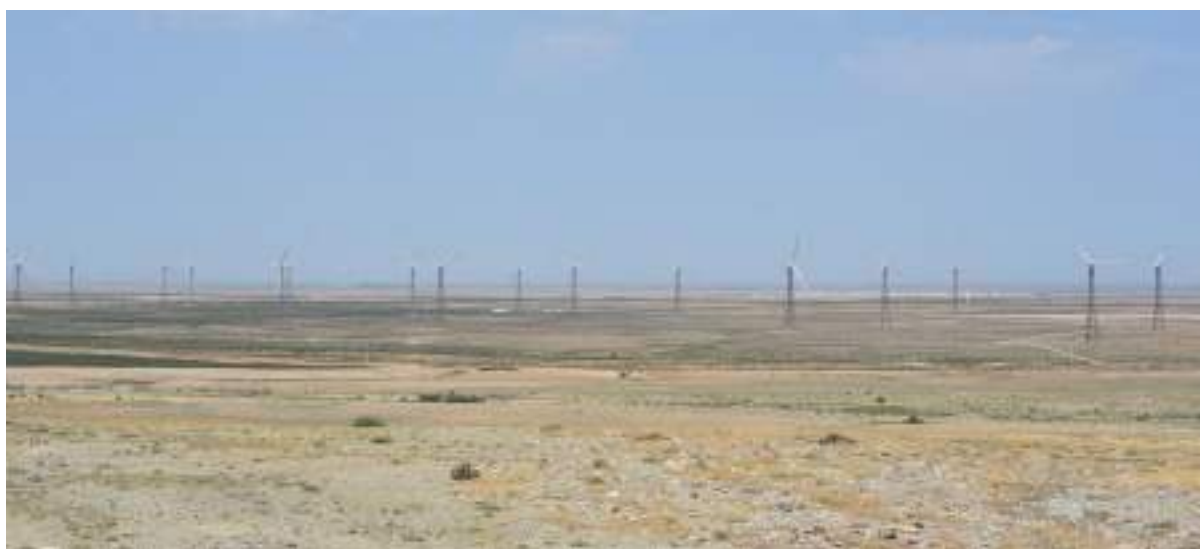
Figure 12-9 Existing Wind Farm
