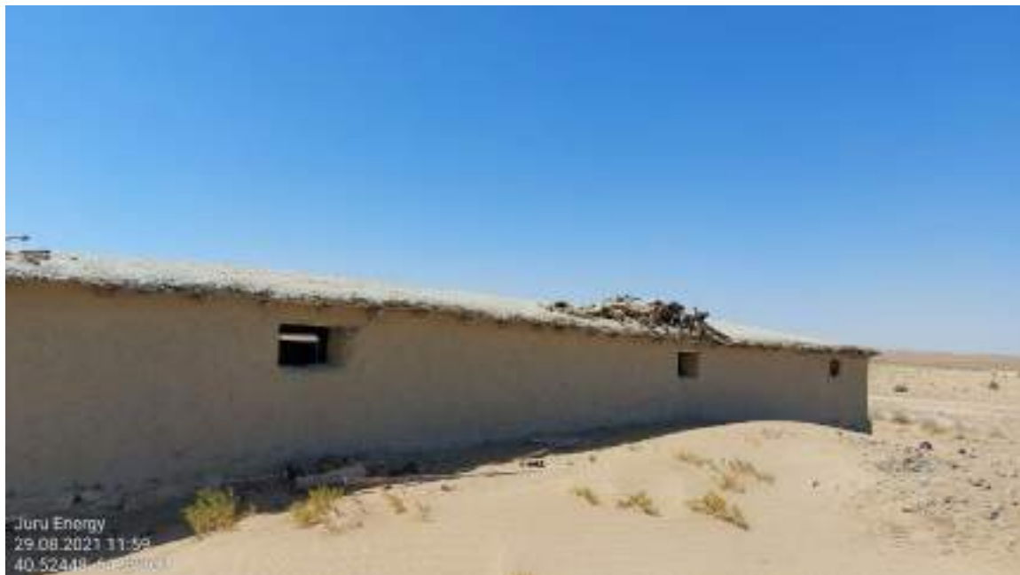
Plate 7-11 Dead Sheep being dried on the roof of a herder's structure (August 2021)
