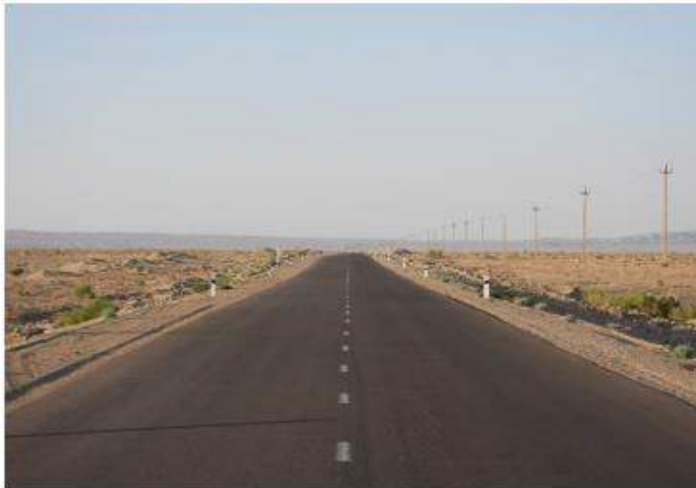
Figure 2-22 View of External Asphalt Road Connecting to Highway A380
