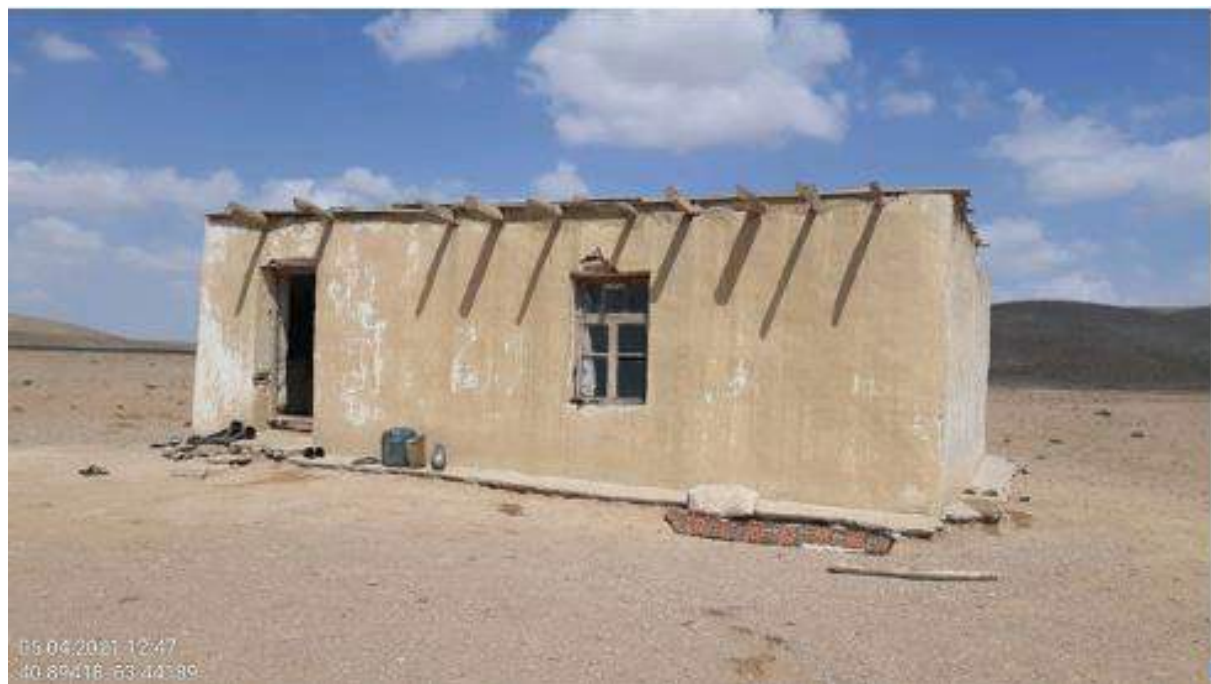
Plate 2-8 View of the Active Settlement – Eastern Plot (April, 2021)
