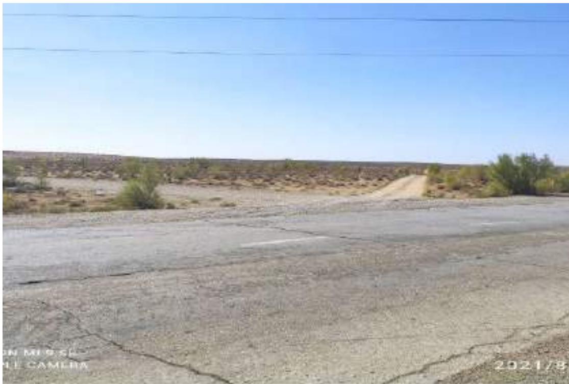
Figure 11-5 View of the Access Road Connecting the Project Site to Highway A379
