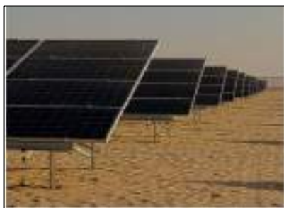
Fixed-tilt mounting system
