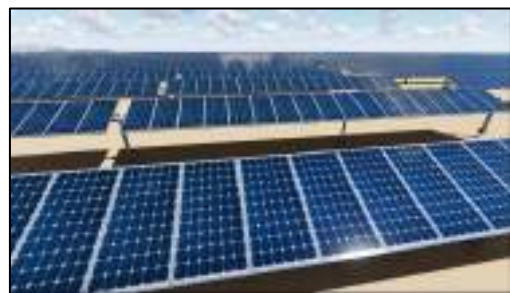
Single-axis tracking system
