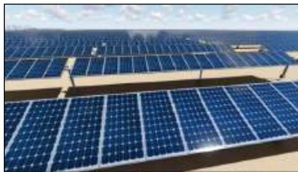
Single-axis tracking system
