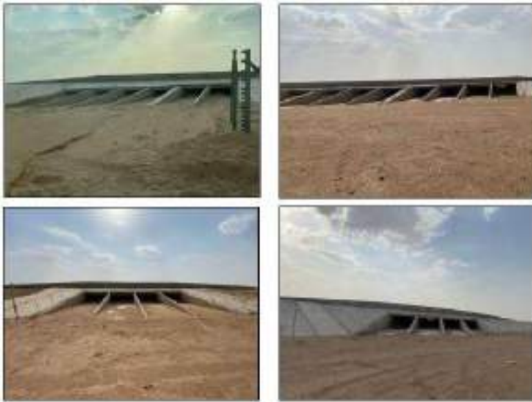
Figure 19 Culverts located along the western site border
