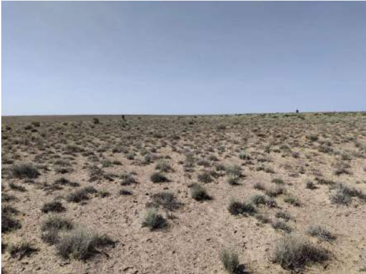
Figure 3. Landscape of wind power plant construction site
