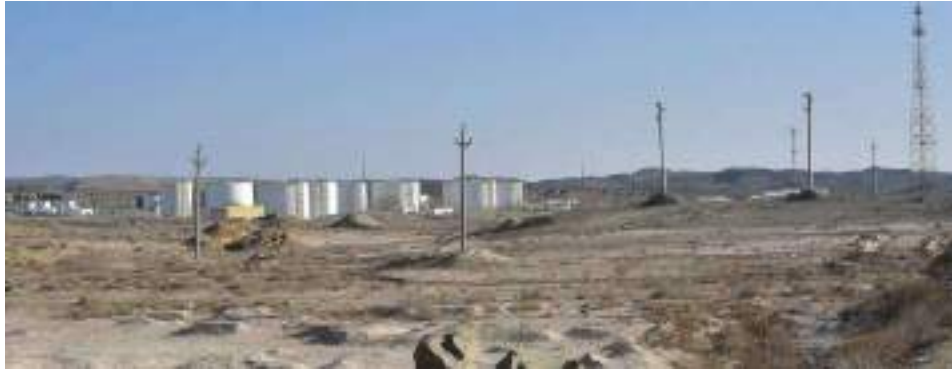
Figure 5-30 Oil Storage Facility
