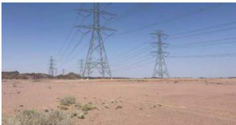
Figure 4.62. Electric tower and line in the project site.
