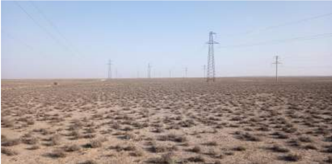
Figure 6 Transmission line locates in Artemisia desert
