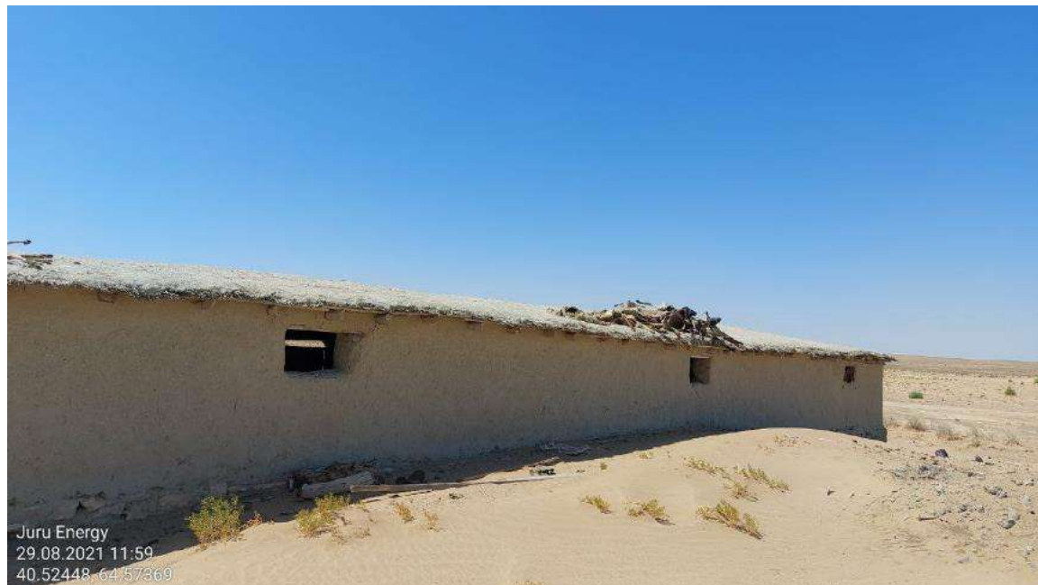
Plate 7-12 Dead sheep being dried on top of the roof
