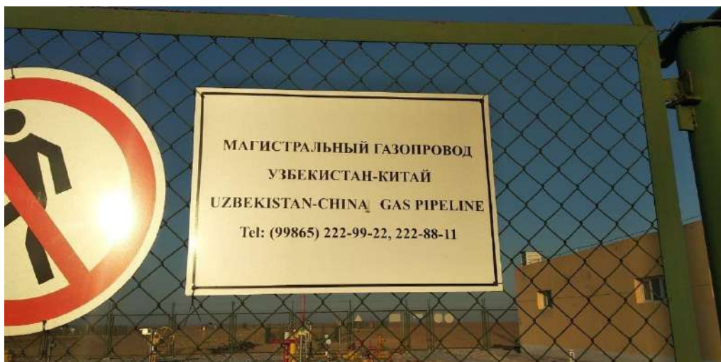
Plate 12-1 Gas facilities at the project site
