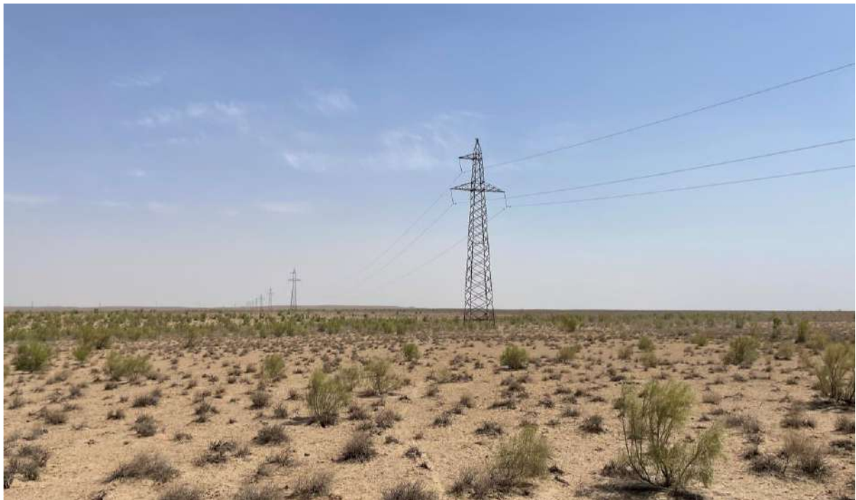
Plate 14-2 Existing Overhead Transmission Lines
