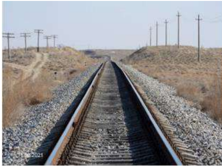
Plate 10-2 View of the Railway Line
