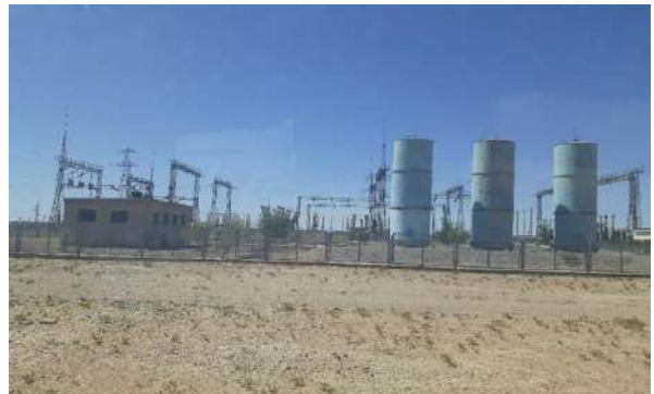
#R13 – View of the Sub-station from the Access Road
