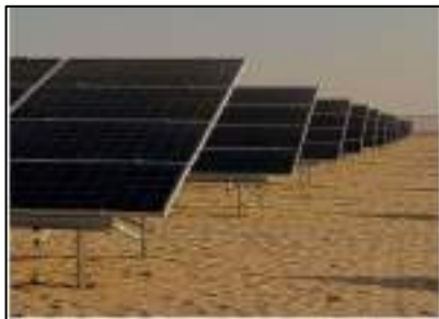
Fixed-tilt mounting system
