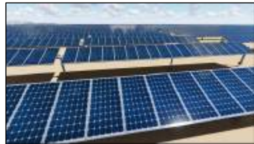
Single-axis tracking system
