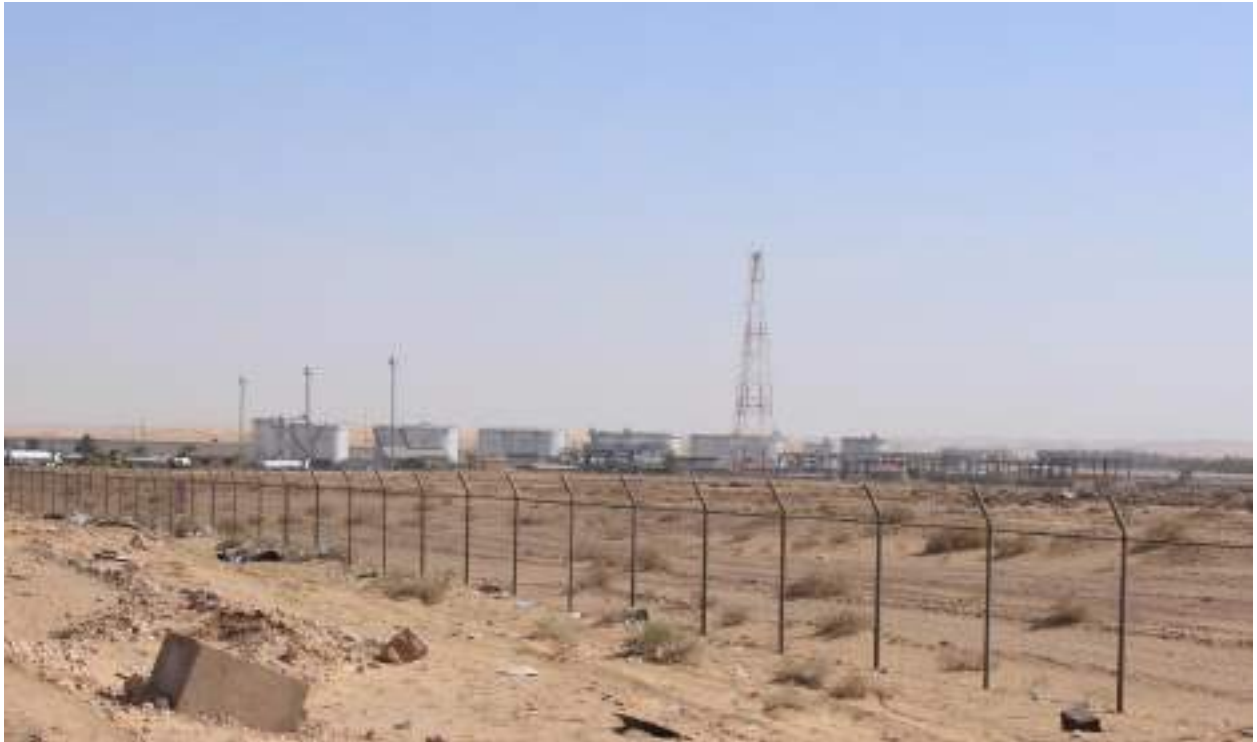
Figure 15-2: Al Jouf Bulk Plant
