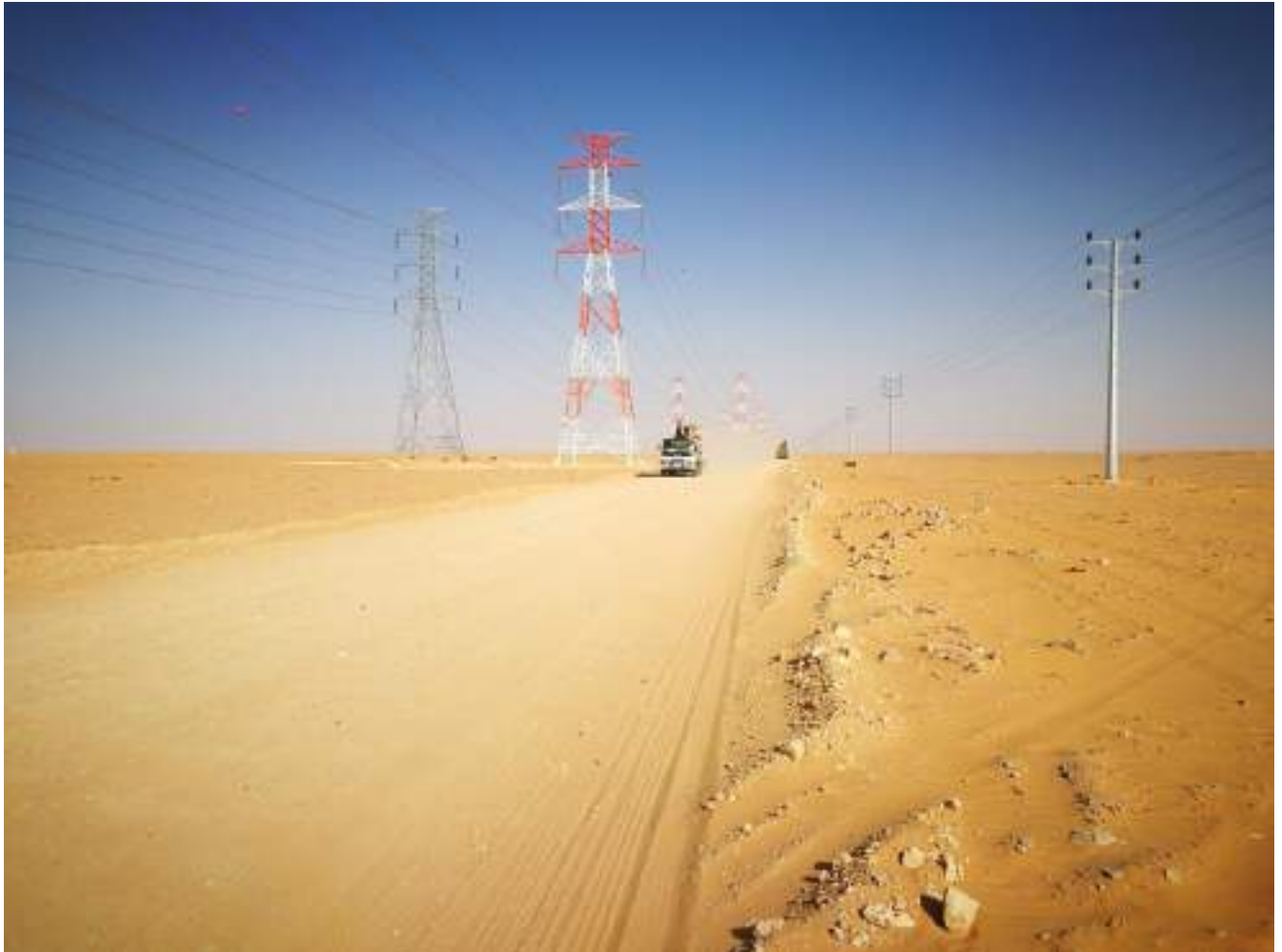
Figure 15-3: 132kV (left of image) and 13.8 kV (right of image) Power Transmission Lines
