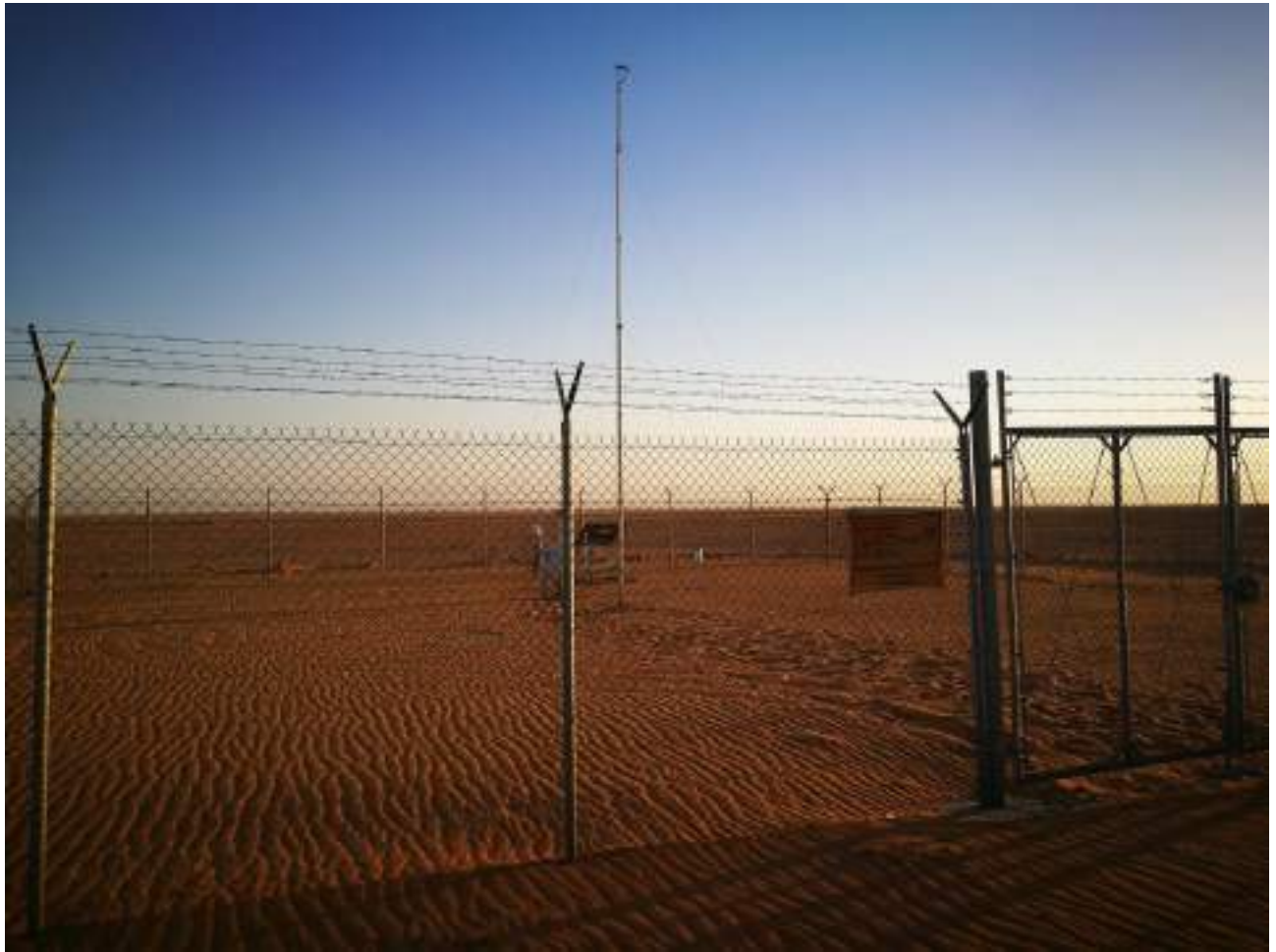
Figure 6-4: Solar Measurement Station
